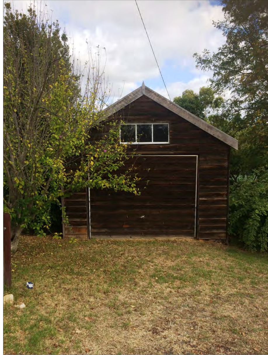
Existing shed in south-eastern corner of 101 Roe Street
